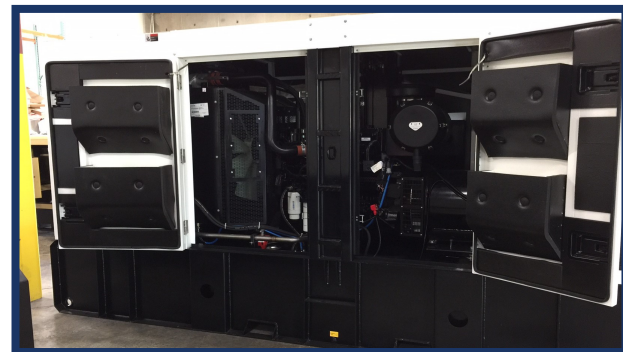
EASY ACCESS FOR MAINTENANCE
